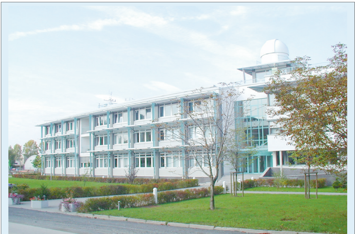
Fig. 1: IFT main building.
